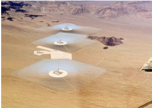
Figure 1 - BrightSource Energy 400MW Ivanpah Plant
